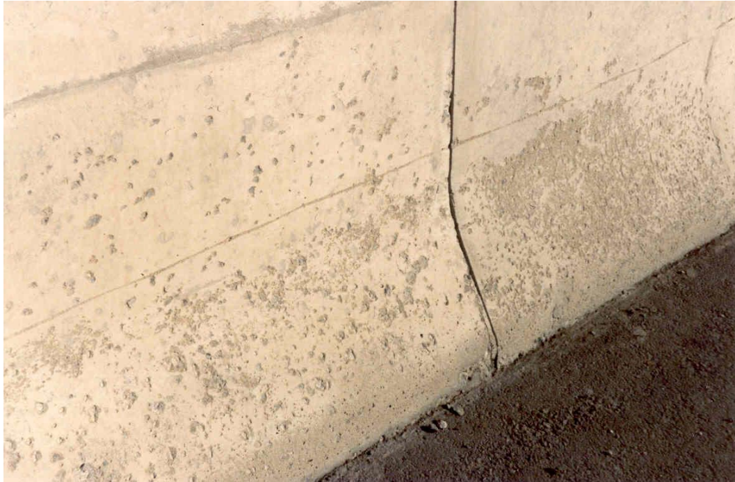
FIGURE 3 Example of Medium Scaling
