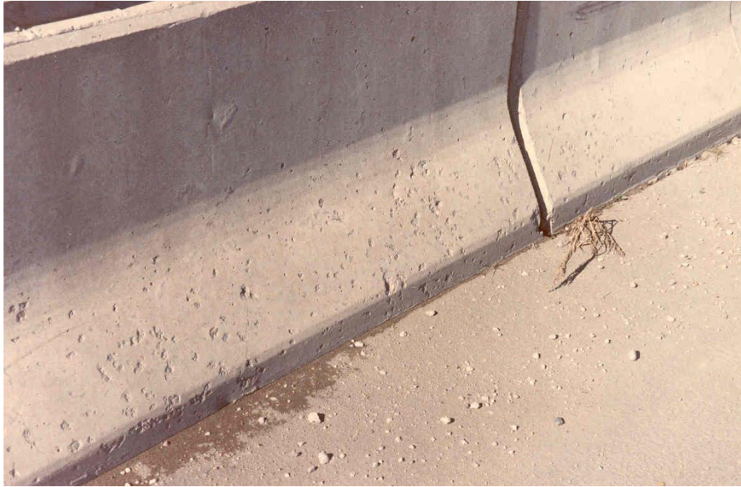
FIGURE 1 Example of Light Scaling
