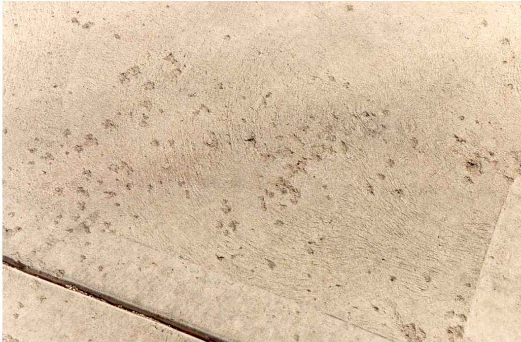
FIGURE 2 Example of Light Scaling
