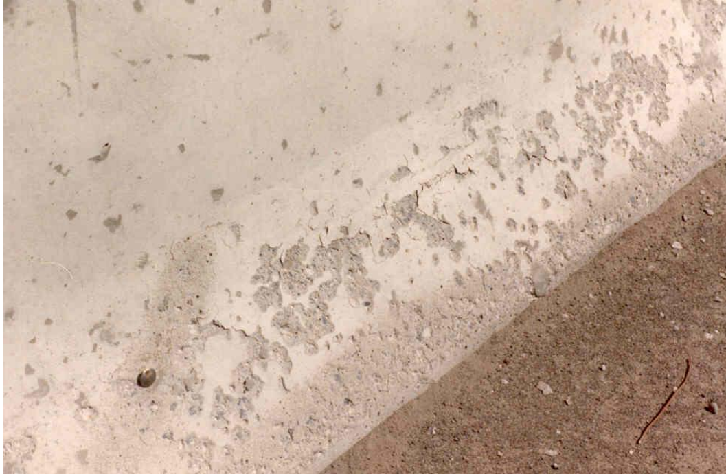
FIGURE 4 Example of Medium Scaling
