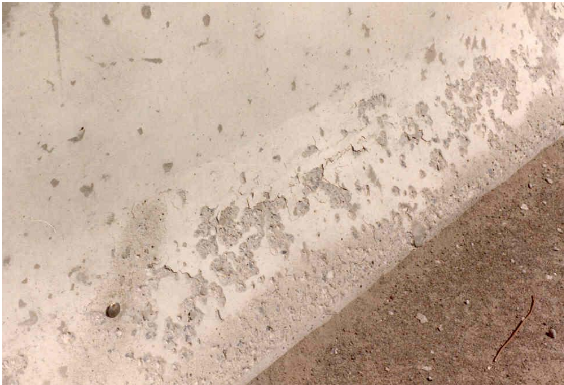
FIGURE 4 Example of Medium Scaling
