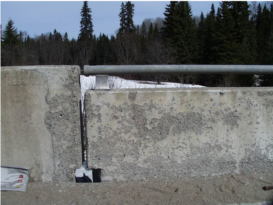
FIGURE 6 Example of Severe Scaling
