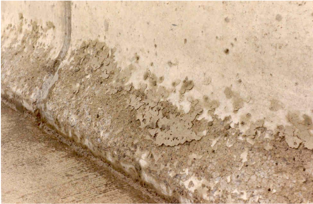
FIGURE 6 Example of Severe Scaling
