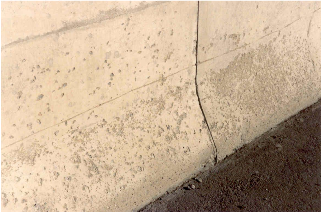
FIGURE 4 Example of Medium Scaling
