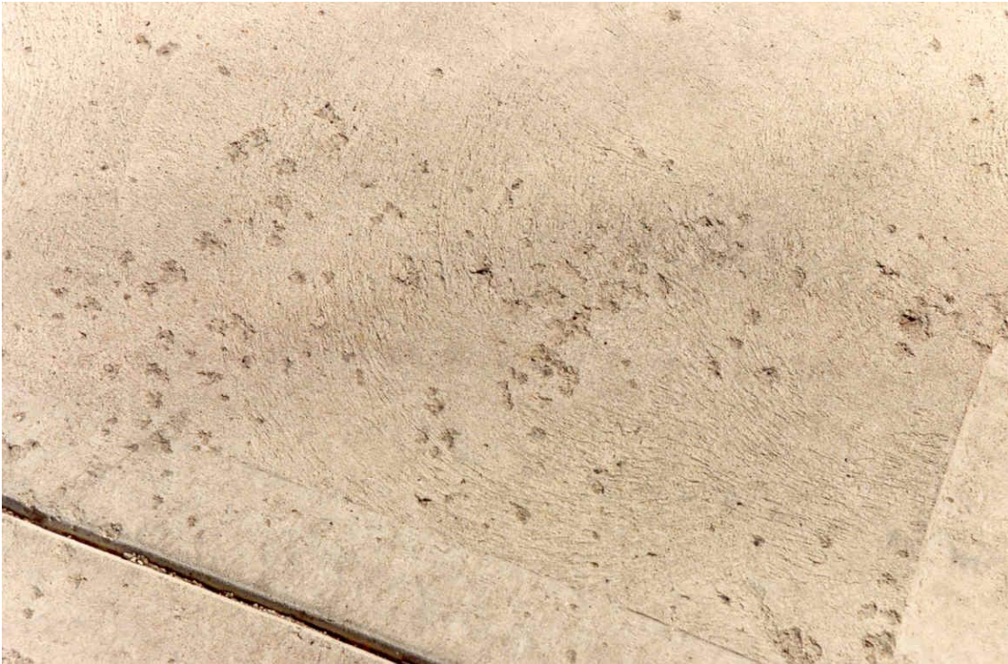
FIGURE 2 Example of Light Scaling
