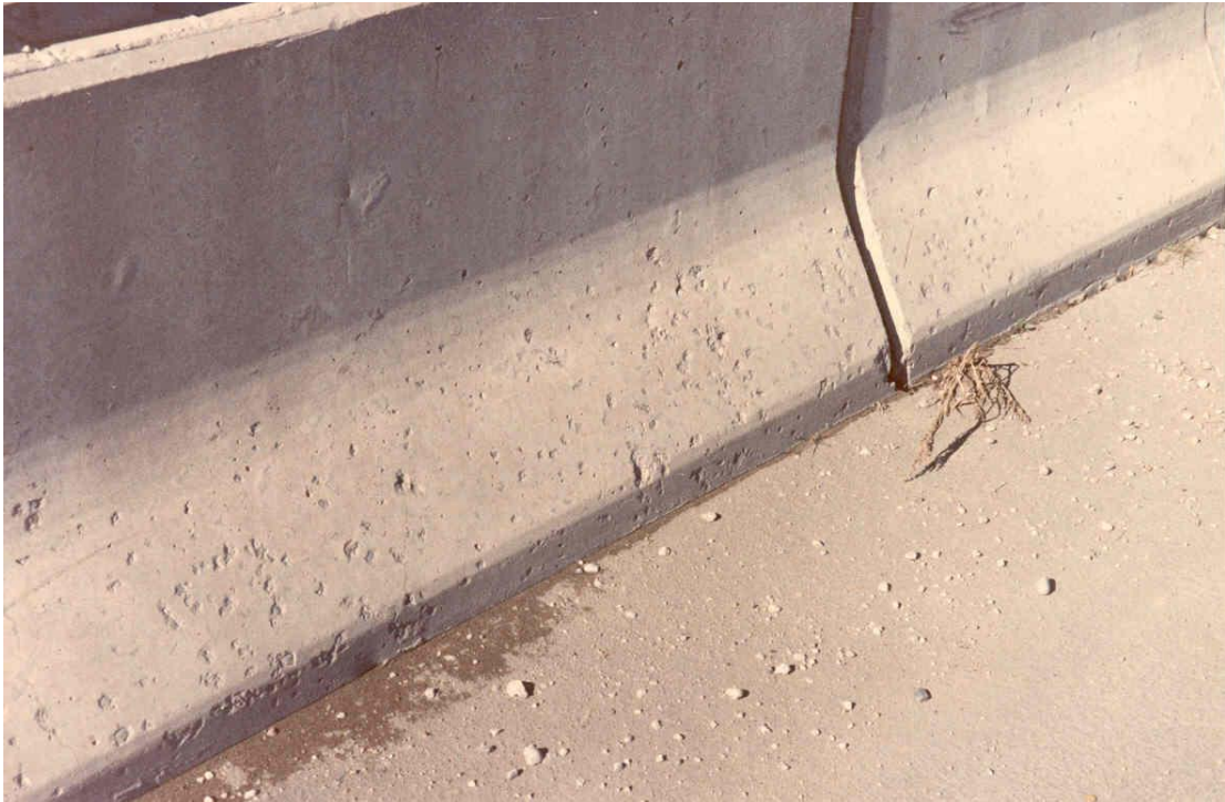
FIGURE 2 Example of Light Scaling
