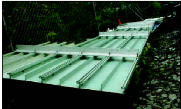
Figure 4.8 – Bolt-together Extruded Panels assembled with T-bars
