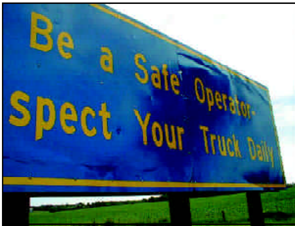
Figure 4.10B Overlay Sheet on Extruded Panel Sign
