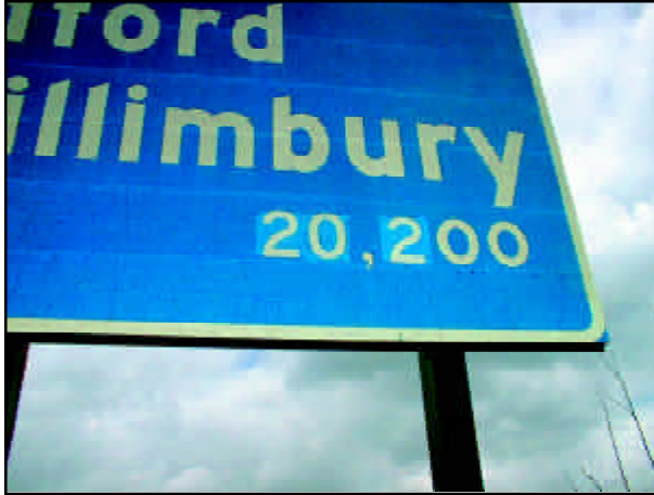
Figure 4.10A Overlay Sheet on Extruded Panel Sign
